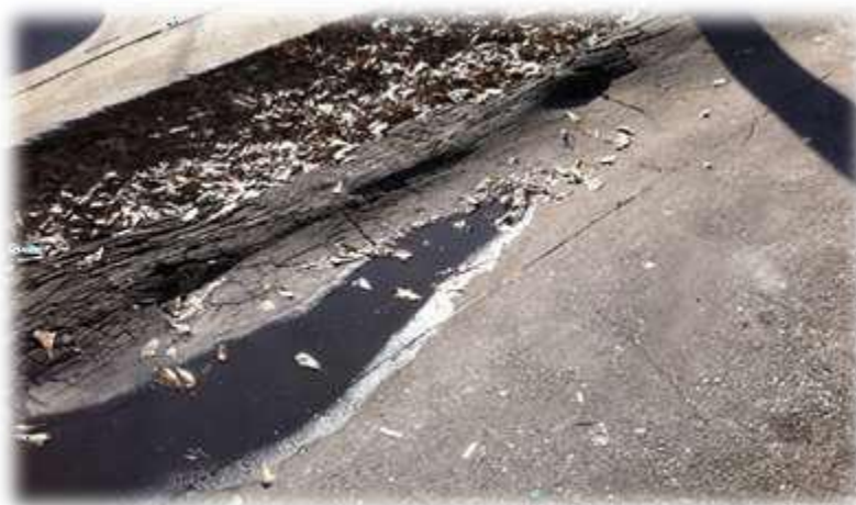
Figure (5) Rutting along the road
