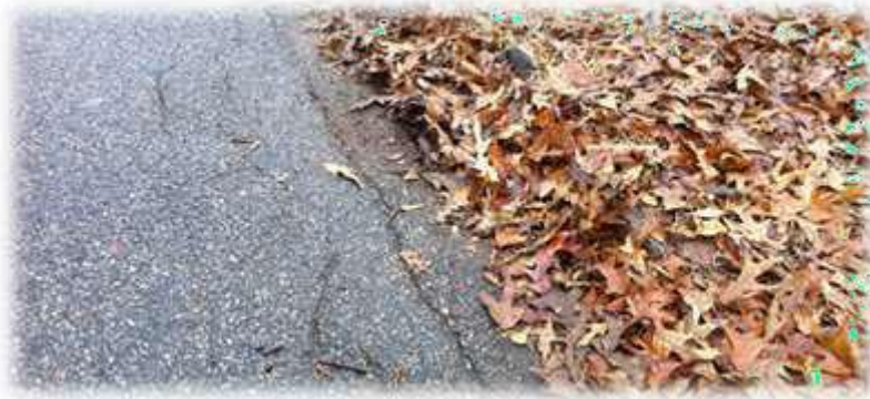
Figure (10) Edge Cracks
