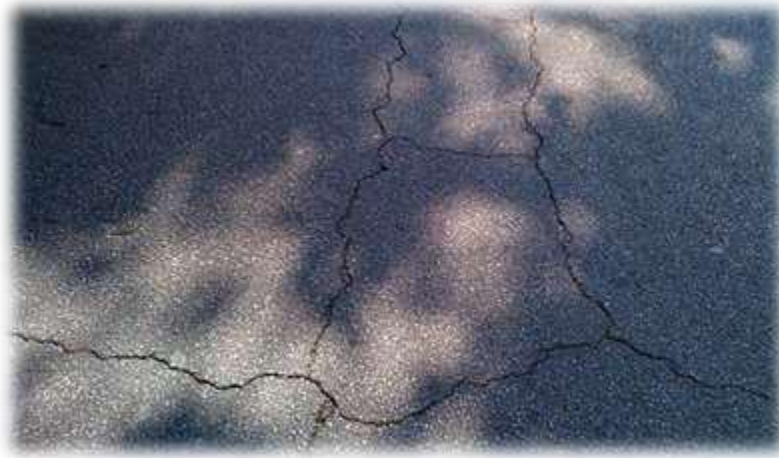
Figure (4) Block Cracking
