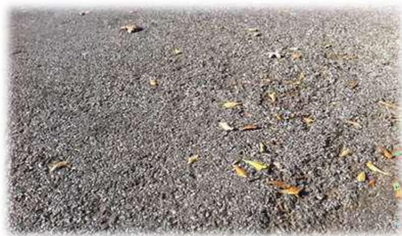
Figure (6) Raveling on the surface
