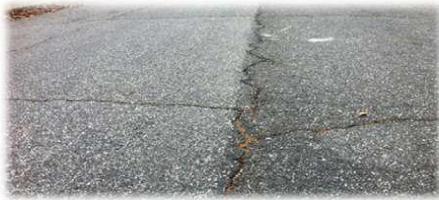
Figure (9) Longitudinal Cracking
