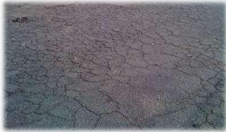
Figure (3) Alligator Cracks on surface
