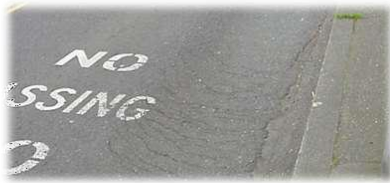
Figure (7) Slippage Cracks
