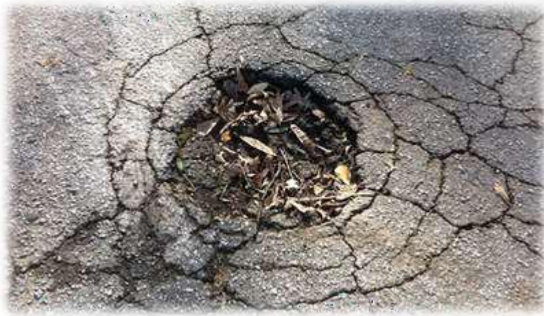
Figure (2) Severe Potholes on Road's Surface
