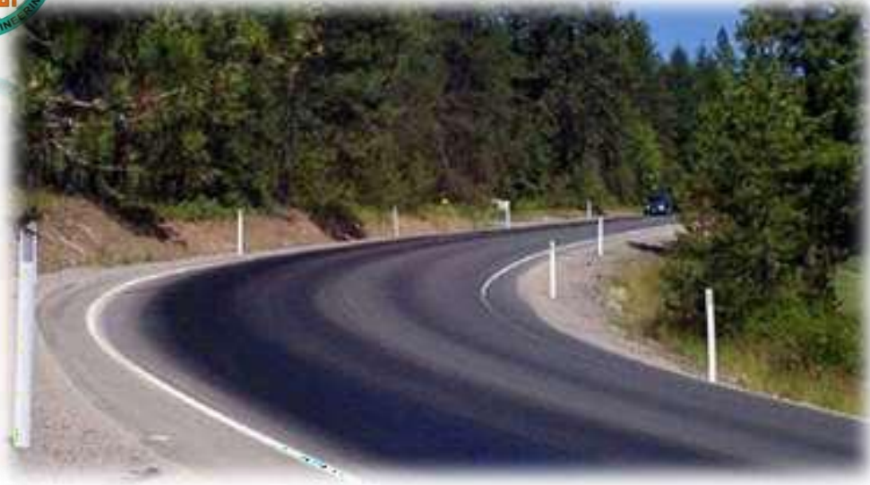
Figure (13) Bleeding seen through a road
