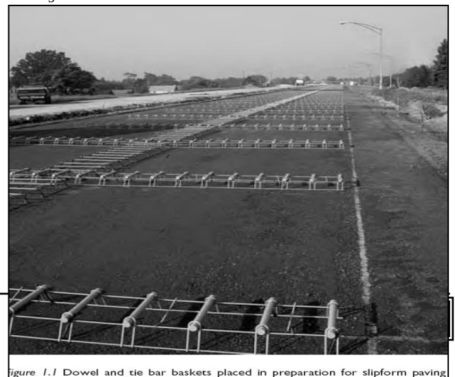
Figure 1.1 Dowel and tie bar baskets placed in preparation for slipform paving
