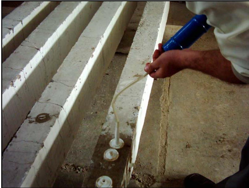
Plate (4) Epoxy injection for beams
