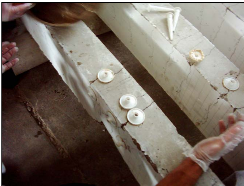
Plate (3) Epoxy injection for beams
